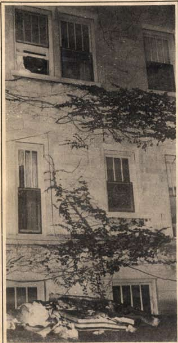
The smoldering mattress and box spring from a fire that campus officials said might have been caused by an over-loaded electrical outlet were dumped out of the second floor Pemberton window Wednesday night by Charleston firemen. (News photo by Brian Ormiston)
